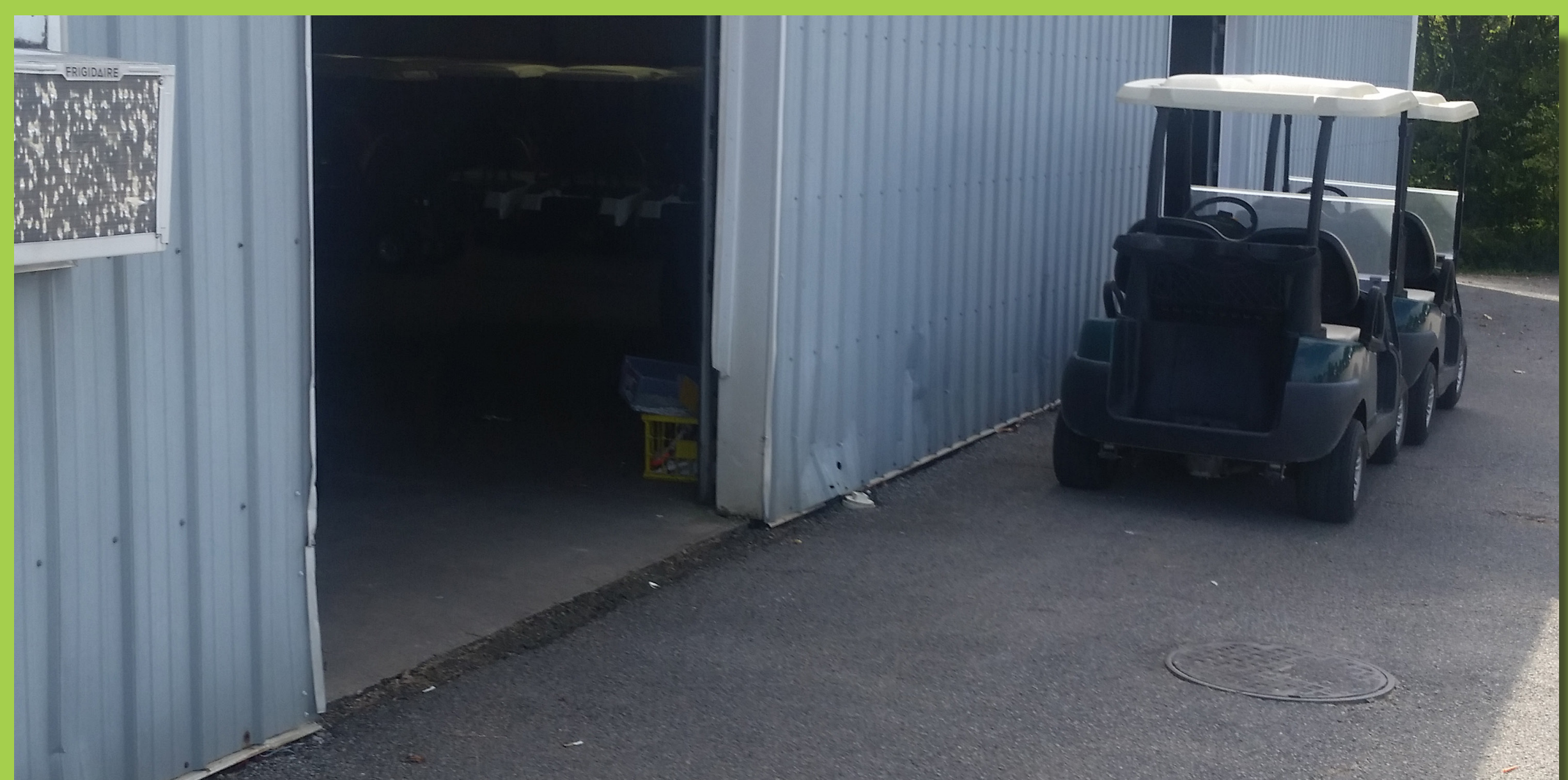
INADEQUATE CART STORAGE
